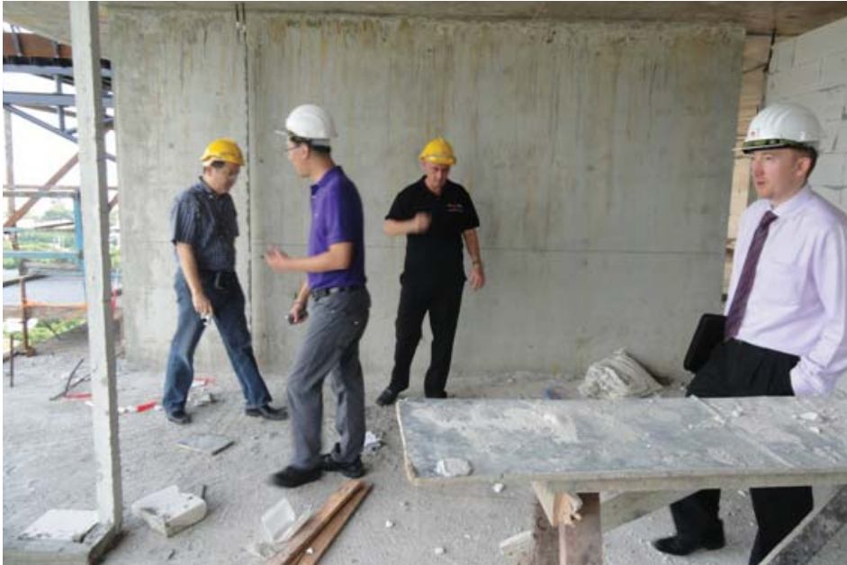
Site inspection at The Cliff, Pattaya
